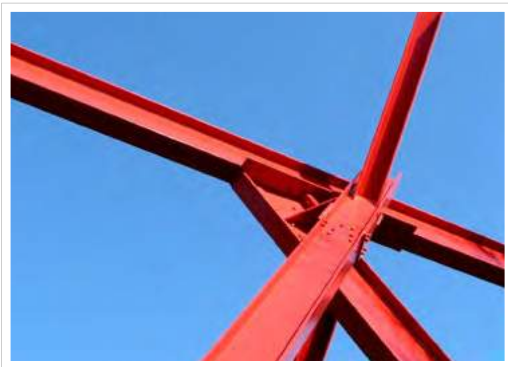
Figure 110. Angles in construction.
